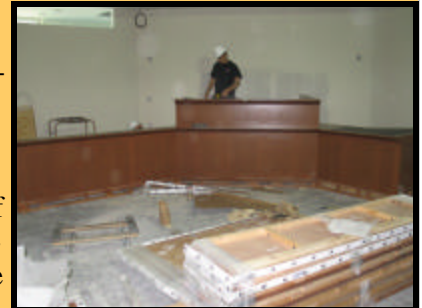
New courtroom under construction
